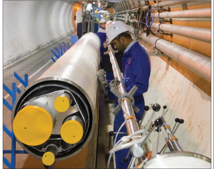
Installation of the cryogenic distribution line on sector 1-2 of the LHC.
