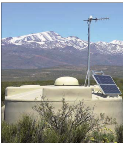
Fig. 3. One of the water tanks in position.
